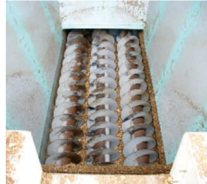
Mounting in discharge screw (wood-fired power plant)
